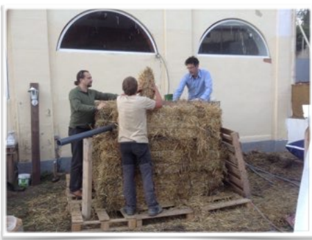
Insulating the Biodigester with straw bales to preserve inner temperatures.
