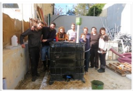
The second Biodigester, built at Arterra during our first public workshop.
